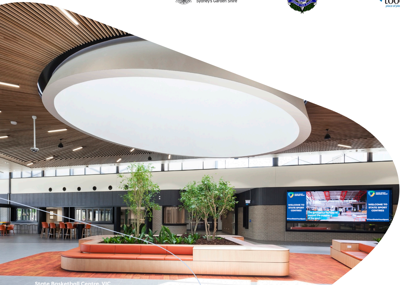
State Basketball Centre, VIC
