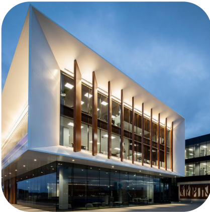
Camden Council Administration Centre
