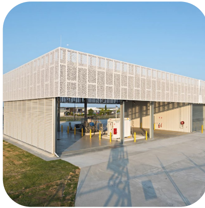
Europcar Facility Sydney Airport
